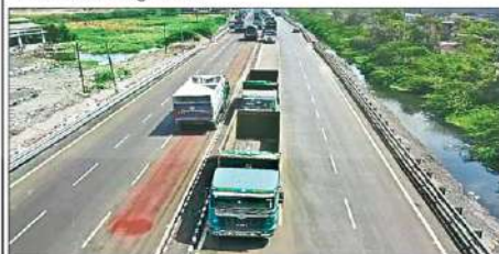
India's First Six-Lane Bituminous Steel Slag Road at Surat, Gujarat
