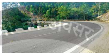
Steel Slag Road in Ziro Valley at Arunachal Pradesh Constructed by BRO over One-Kilometer Stretch
